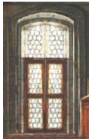
A rectified, front-on view of the window
