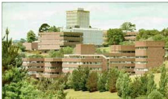
The Physics building tower at Exeter University. (Copyright: Exeter University .)
